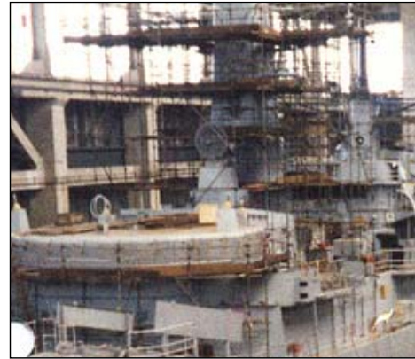
Figure 11: Temporary Staging Erected around Mast for Maintenance
